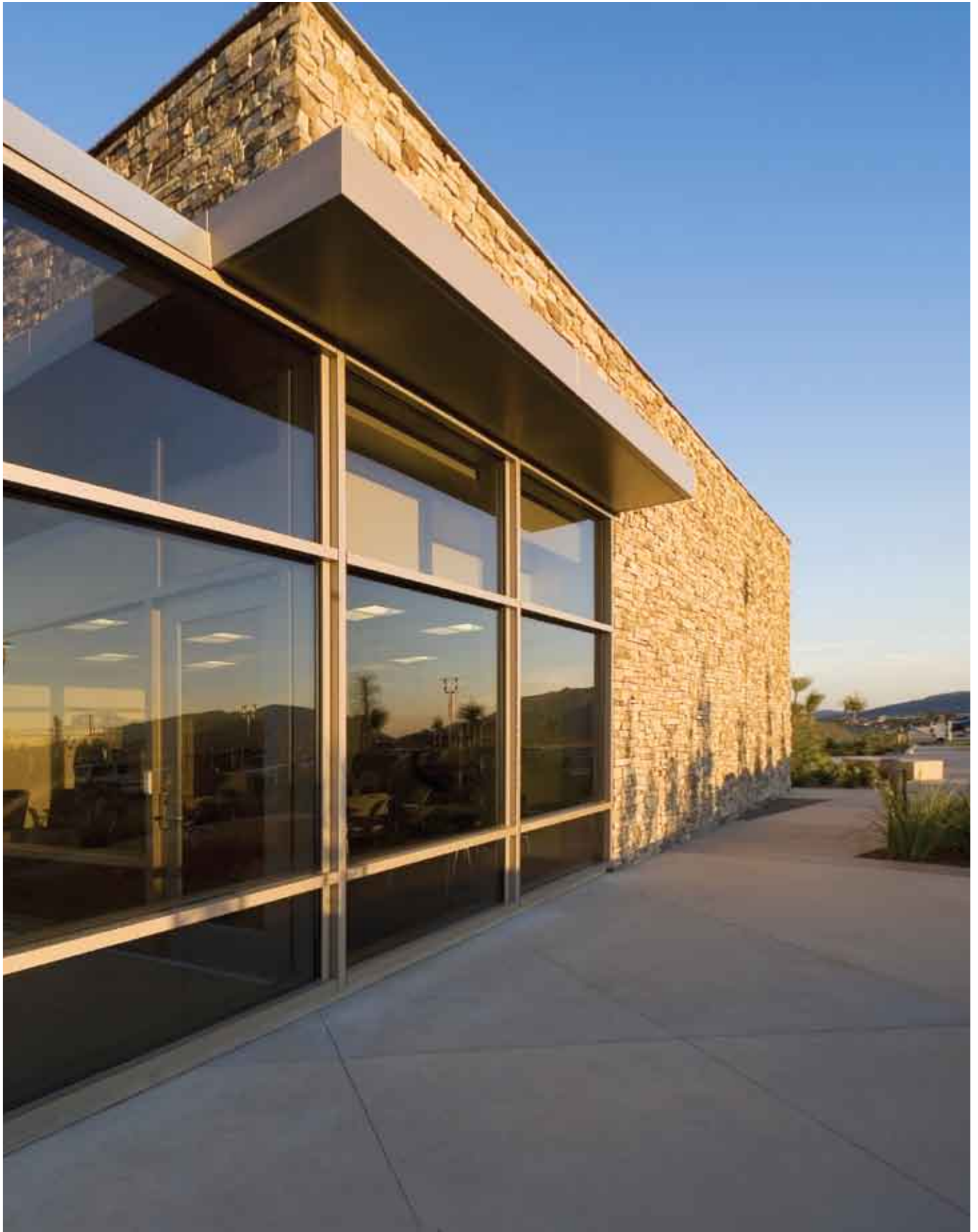
Manzanita Cliffstone with a dry-stack grout technique
