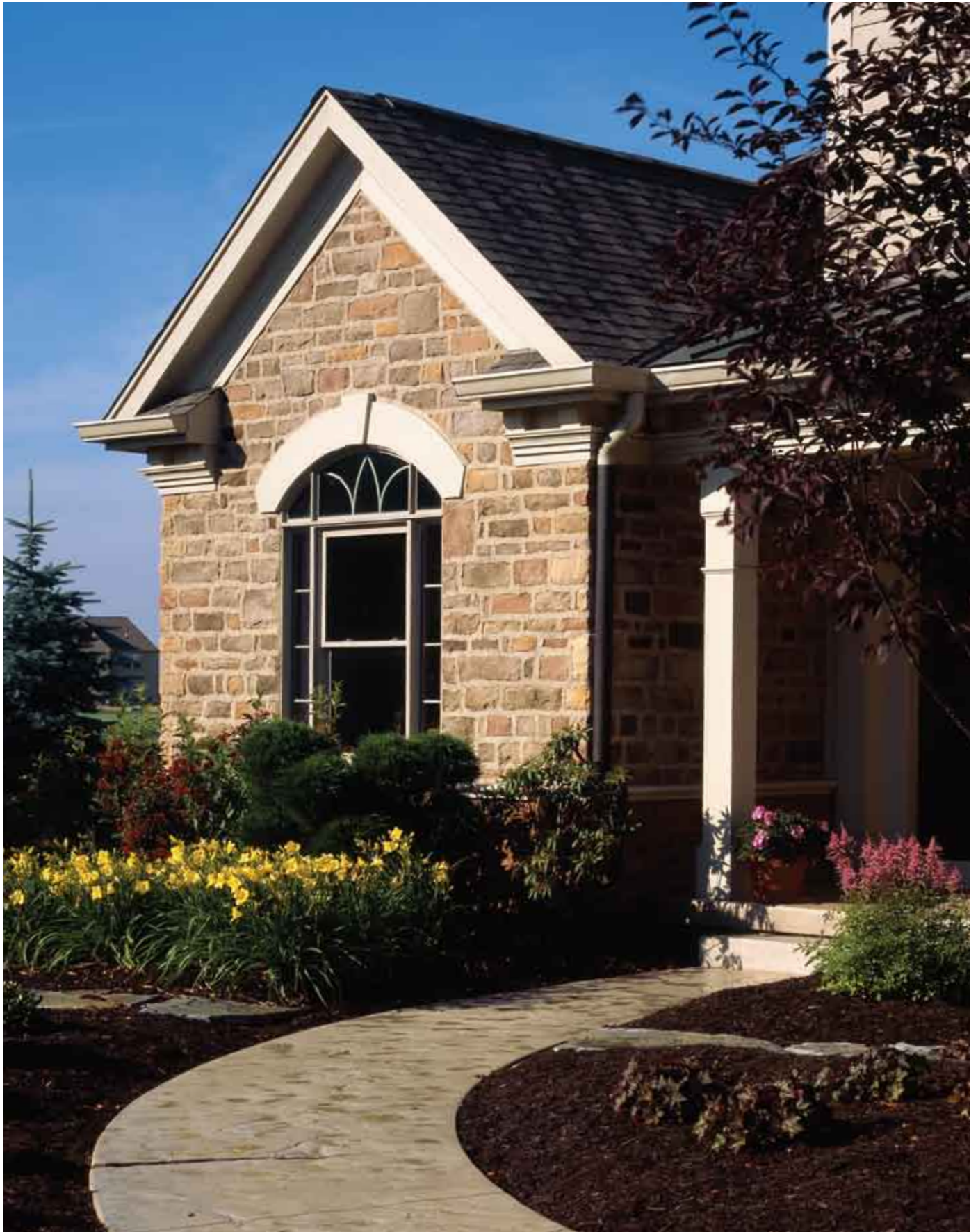
Bridgeport Limestone with an overgrout technique
